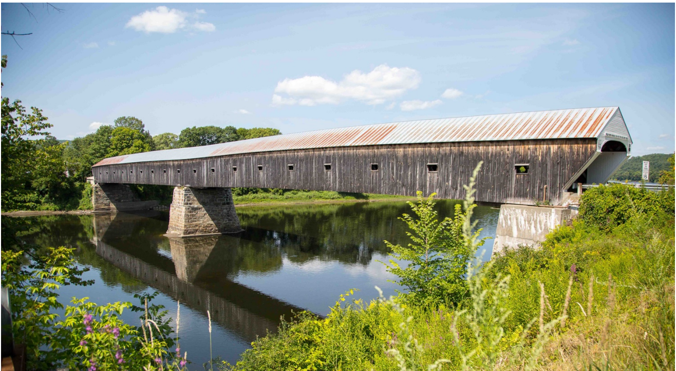
Cornish-Windsor Covered Bridge
