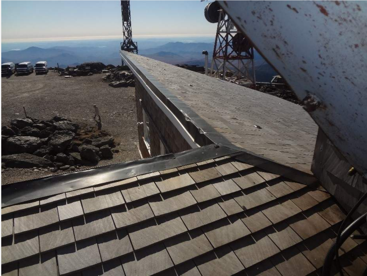
2017 Conditions (Roof Replaced 2019)
