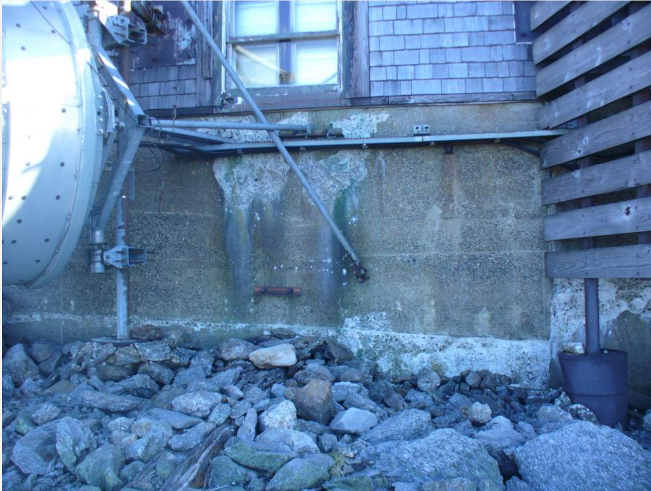
West Facing Foundation
