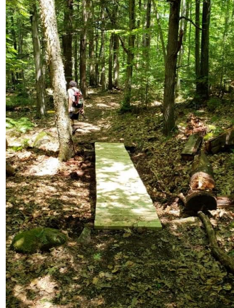
Bridge built by Southern NEMBA on the chipmunk trail at Bear Brook State Park
