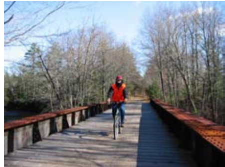
Rail Bridge over Lamprey River
