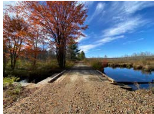
Fitzwilliam Bridge Cheshire Rail Trail
